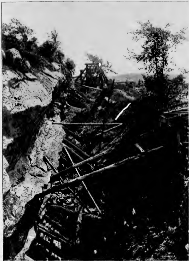
FIG. 85.—View of the west vein at Franklin Furnace looking south. The two shafts are at the Trotter Mine. Photographed by J. F. Kemp, 1893.
